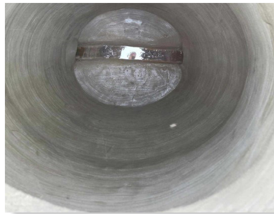
The City contracted with SAK for cured in place sewer rehabilitation and manhole rehabilitation. This prevents further breakdown of sewer line and manholes through a relining process which provides greater structural integrity.
